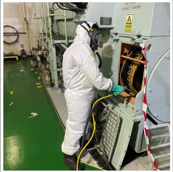
IN-SITU CHEMICAL CLEANING OF ALTERNATOR
