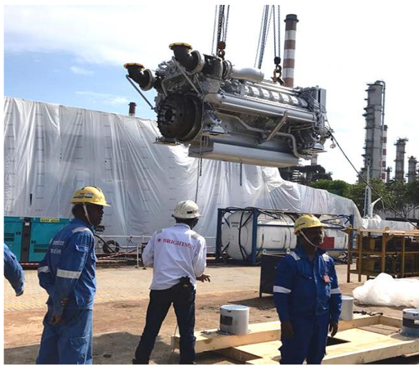
HEAVY LIFTING OPERATION
