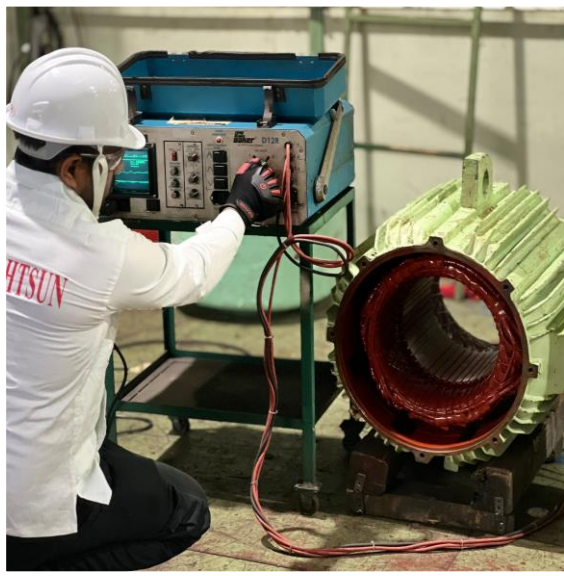
ELECTRICAL MOTOR HEALTH ANALYSIS
