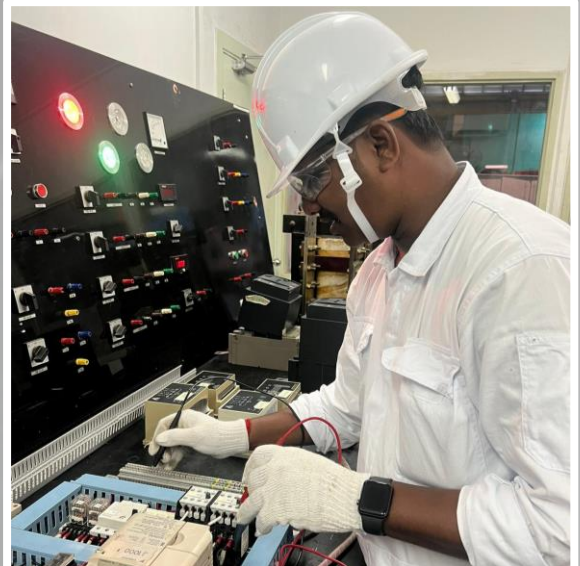
ELECTRICAL INSTRUMENTS TESTING LAB
