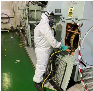
IN-SITU CHEMICAL CLEANING OF ALTERNATOR
