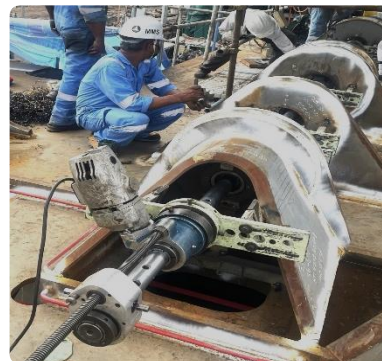
IN-SITU BORING WORK
