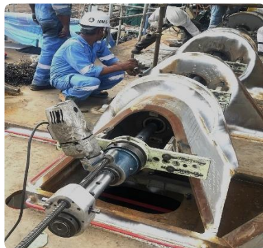
IN-SITU BORING WORK
