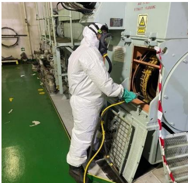
IN-SITU CHEMICAL CLEANING OF ALTERNATOR
