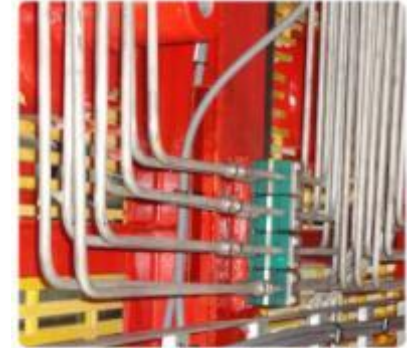
PIPE TUBING RENEWAL
