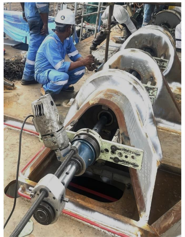
IN-SITU LINE BORING
