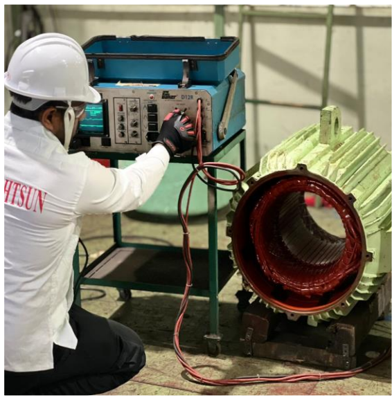
ELECTRICAL MOTOR HEALTH ANALYSIS
