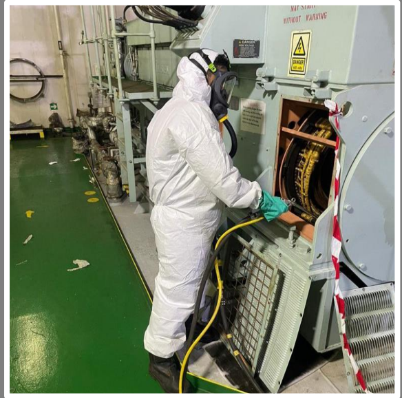
IN-SITU CHEMICAL CLEANING OF ALTERNATOR
