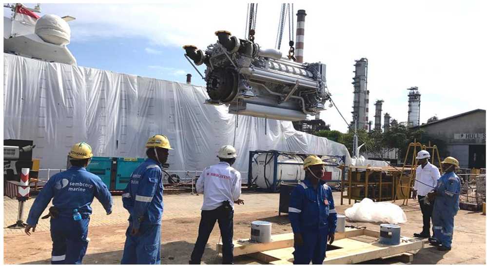
HEAVY LIFTING OPERATION
