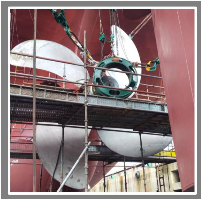
PROPELLER & TAIL SHAFT INSTALLATION
